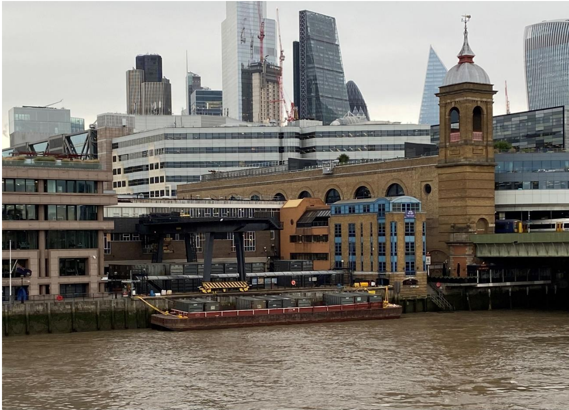
Figure 2: Walbrook Wharf, view from southwest
